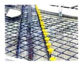
In this scenario, if a top layer of rebar (mat) is required in the design, it is impossible to tie the upper mat to the vertical rebar without removing the protective caps and covers. But if the protective caps and covers are removed while the upper mat is actively being constructed, the worker positioning and tying the upper mat of rebar will be exposed to the impalement hazard presented by the rebar protruding from the lower layer.
